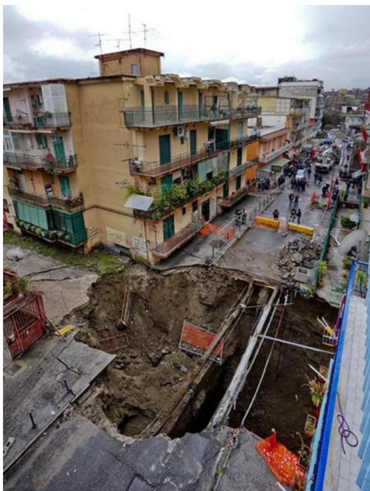
Figure 11. The sinkhole on Via Campanile, in the Pianura neighborhood of Naples. Image source: ANSA (2015), “Voragine a Napoli, causa rottura condotta”. [22]
