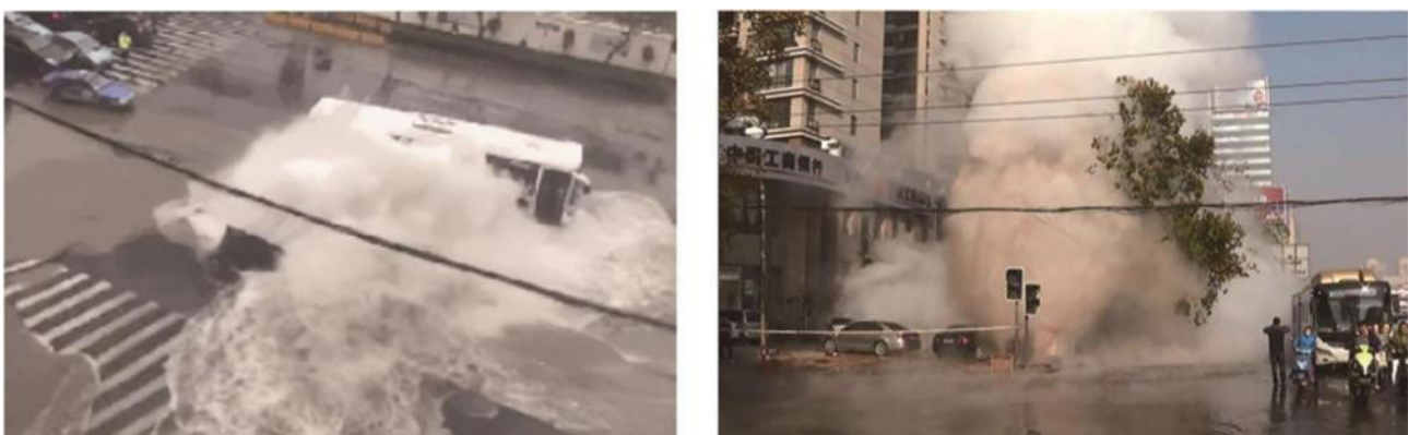
Figure 7. Reproduced from Chao et al. (2025) [18]. Two typical urban pipe burst accidents: on the left, the event in Shanghai, China (November 11, 2017); on the right, the event in Zhengzhou, China (December 6, 2013).
