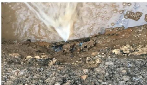
Corrosion pin hole on an iron pipe.
